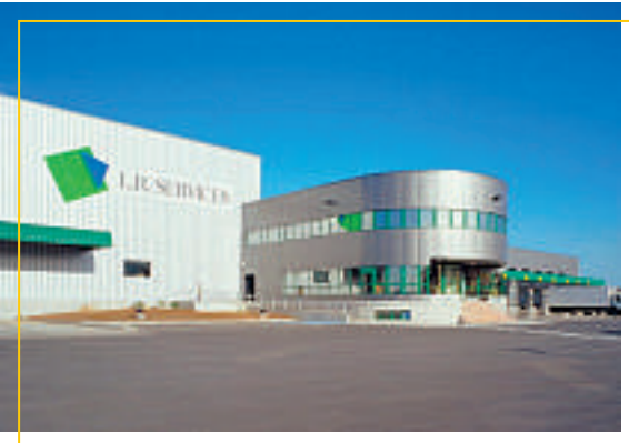
Cold storage, France
