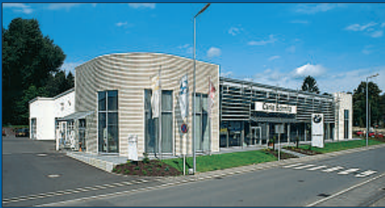
Luxembourg - Showroom and garage
